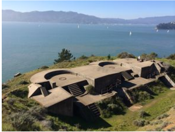
Battery Ledyard, near Point Knox, was active between 1899 and 1915.
